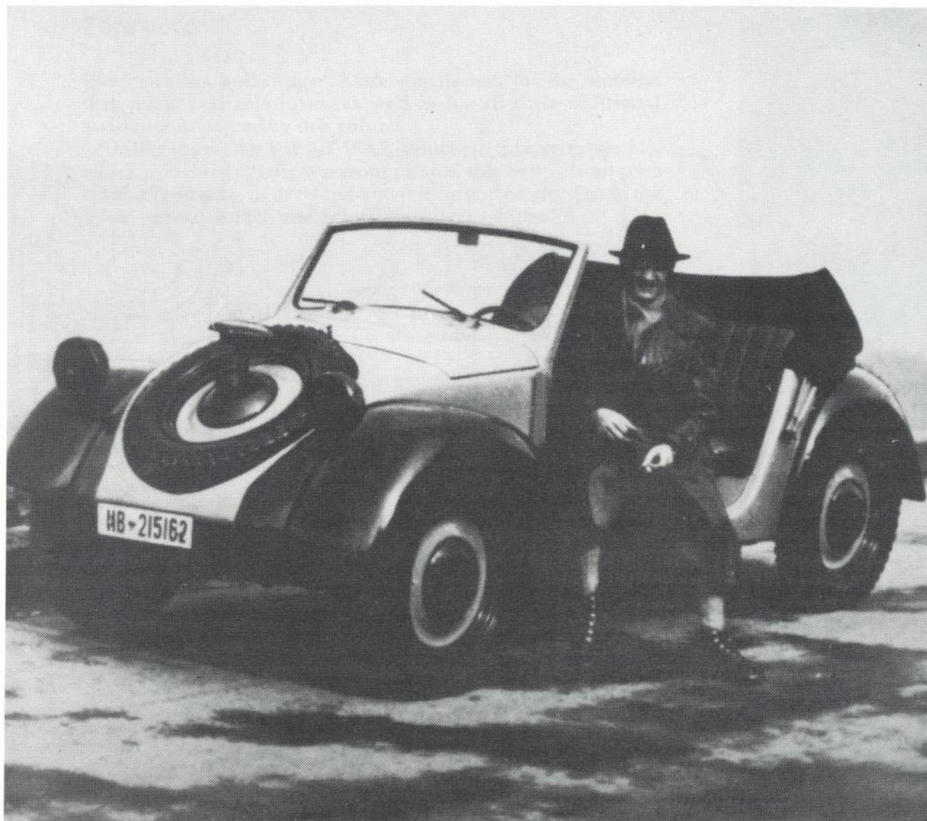
The first model of the VW Kübelwagen Type 62. The body still resembles that of the Beetle or its convertible version. This styling did not suit the military, as it looked too civilian.
